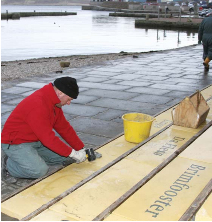
Stonemason Bruce Clubb laying the new pavers.
